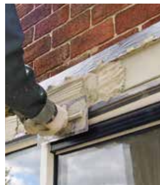
Belzona 4141 (Magma-Build) Lightweight epoxy concrete repair mortar suitable for vertical and overhead applications.
