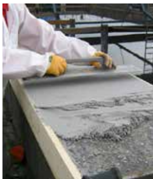
Belzona 4131 (Magma-Screed) Epoxy impact and abrasion-resistant concrete repair mortar.
