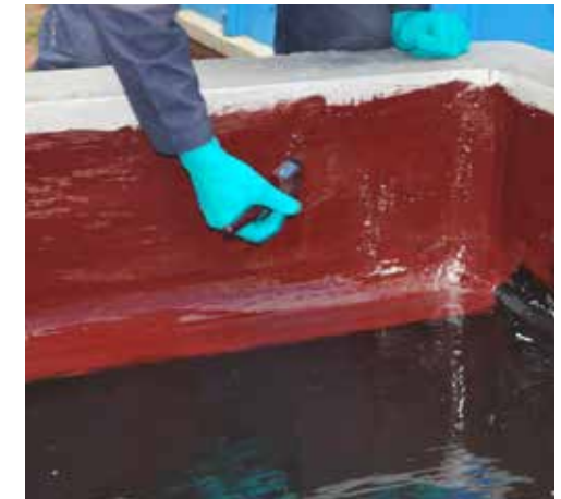
Belzona 4361 Flexible chemical-resistant epoxy barrier coating suitable for concrete protection. Particularly suitable for areas subject to movement.
