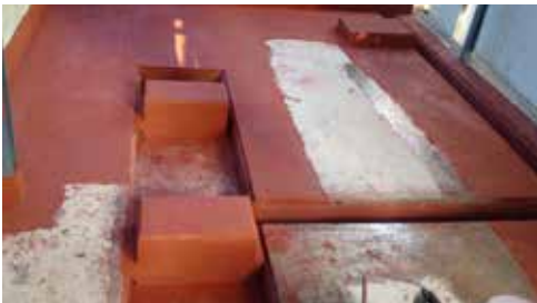
Belzona 4181 (AHR Magma-Quartz) Acid and heat-resistant epoxy concrete repair mortar.
